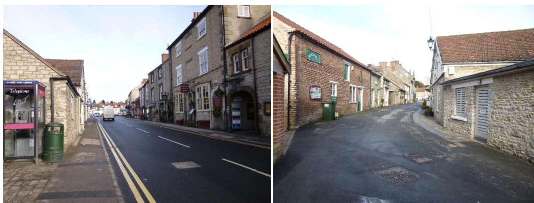
Commercial Area of Helmsley
